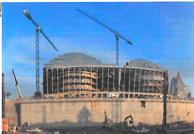
Instead of cables, slightly larger hot-rolled steel tension rods (visible in the foreground) are providing fire safety at the Kauffman Center for the Performing Arts, under construction in Kansas City, Mo., without the need to apply additional protective material.
